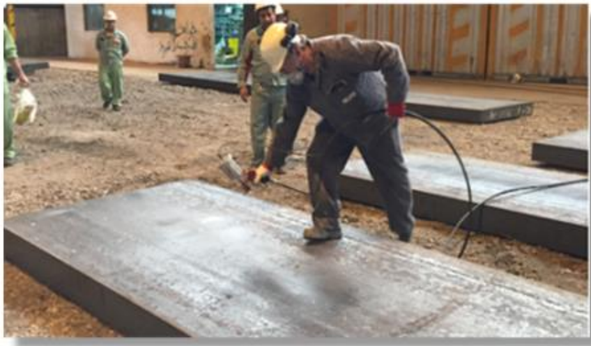
Figure 12 : Application of protective coatings
