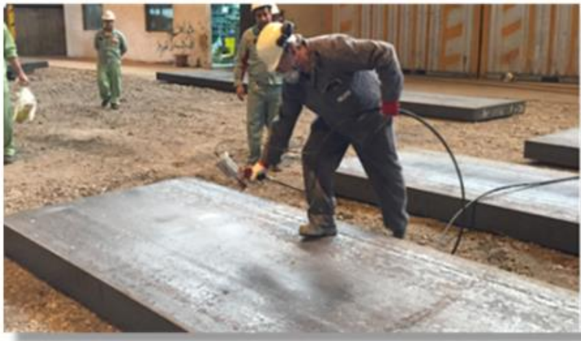
Figure 42: Application of protective coatings
