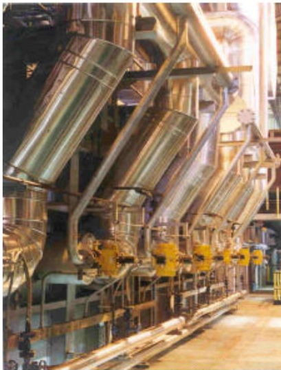
Figure 23: Installation of burners
