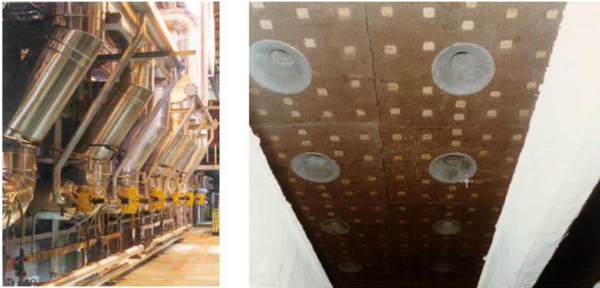
Figure 4 : Installation of burners
