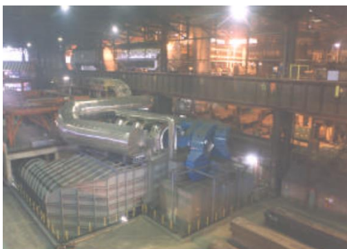
Figure 5 : Heat recuperators
