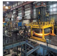
Scrap processing and electric steelmaking plants
